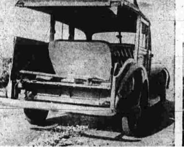
Here's the job completed. New corner posts, siderails and panels plus new tail gate and top. Your Station Wagon needs the same high type work and materials as a good boat.
